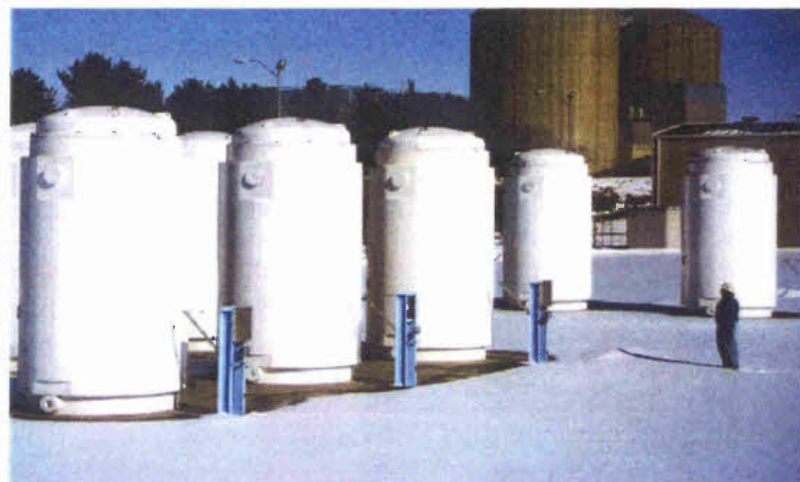
Figure 15-25 After 3 or 4 years in a reactor, spent-fuel rods are removed and stored in a deep pool of water contained in a steel-lined concrete basin (left) for cooling. After about 5 years of cooling, the fuel rods can be stored upright on concrete pads (right) in sealed dry-storage casks made of heat-resistant metal alloys and thick concrete. Questions: Would you be willing to live within a block or two of these casks or have them transported through the area where you live in the event that they were transferred to a long-term storage site? Explain. What are the alternatives?
