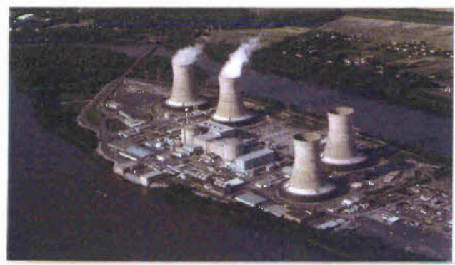
Figure 15-22 This water-cooled nuclear power plant, with a pressurized water reactor, produces intense heat that is used to convert water to steam, which spins a turbine that generates electricity. Question: How does this plant differ from the coal-burning plant in Figure 15-15?
